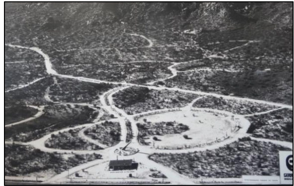
Carefree Village Center (1959) – This aerial image displays the original natural setting of the Village Center and the prevalence of a well-defined two-lane divided main entry drive that connects directly to the sundial in the foreground.
