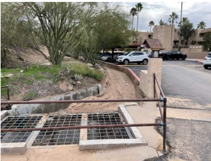
Photo 2 – Drop Inlet Structure to 42-inch Storm Drain (Looking Southeast)
