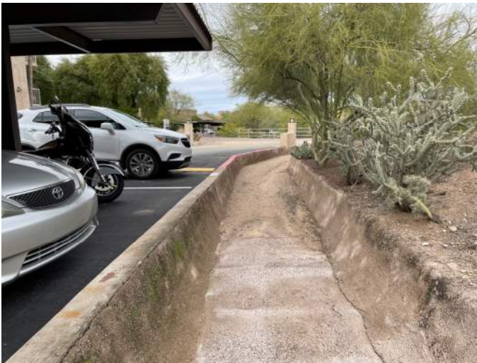
Photo 1 – Trapezoidal Shotcrete Lined Channel (Looking Northwest)
