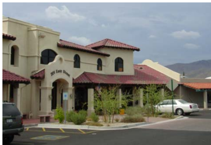
Multiple roof forms
